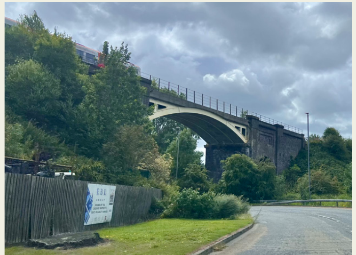
↑ View from Clifton Road of the Mid-Cheshire Railway Line into Frodsham
